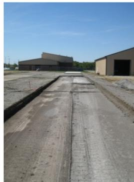
Figure 10. Milled asphalt concrete.
