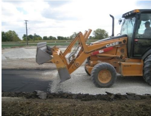
Figure 11. Granular base over geotextile.
