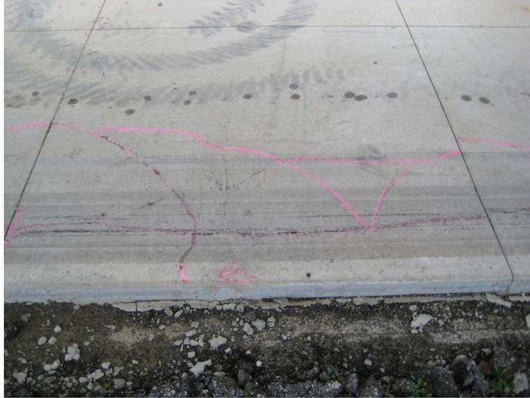
Figure 94. Fatigue cracking of 4 in. concrete slab over asphalt base on section 1 south at 56 million ESALs.
