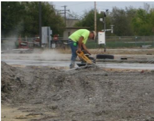
Figure 16. Manual saw cutting of edges.
