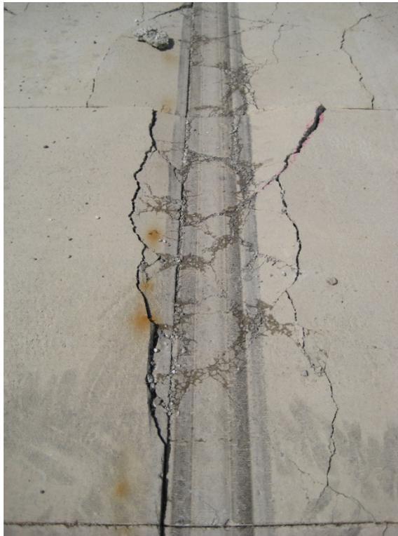
Figure 98. Longitudinal joint on 3.5 inch FRC section.
