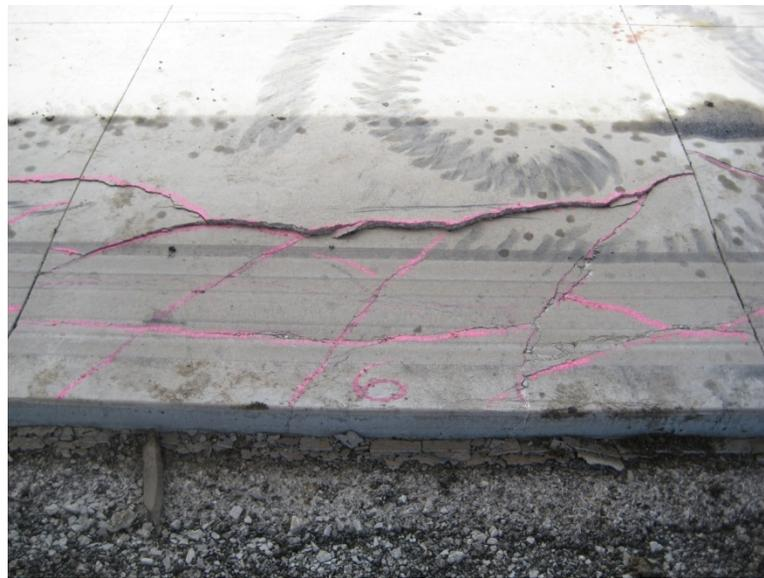
Figure 93. Fatigue cracking of 4 in. concrete slab over asphalt base on section 1 north at 20 million ESALs.
