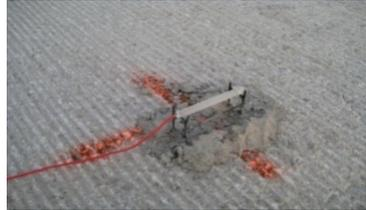
Figure 9. Strain gauge on steel chair prior to paving.
