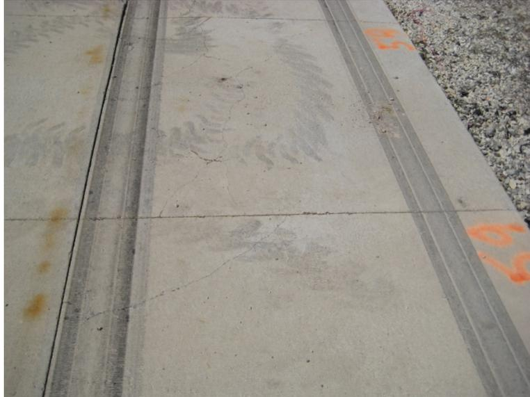
Figure 97. Longitudinal joint opening on 3.5 inch plain concrete section.
