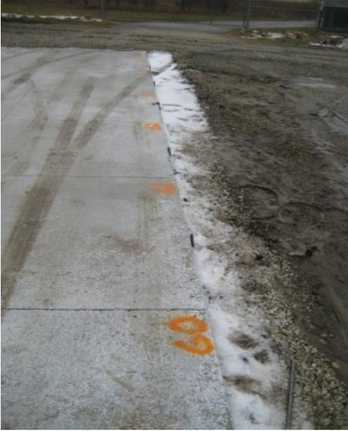
Figure 17. Lateral restraint pins.
