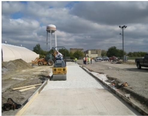
Figure 12. Compaction of granular base.
