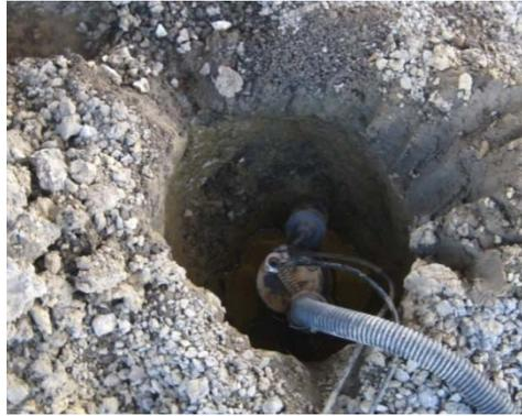
Figure 57. Water pump used to drain Section 2 North.
